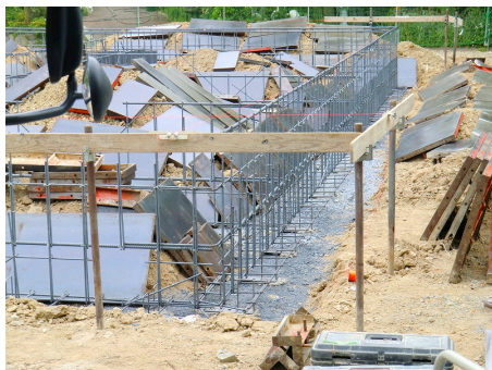
Fig. 1. Groundwork of a building: an assembling cage for reinforced-concrete.
