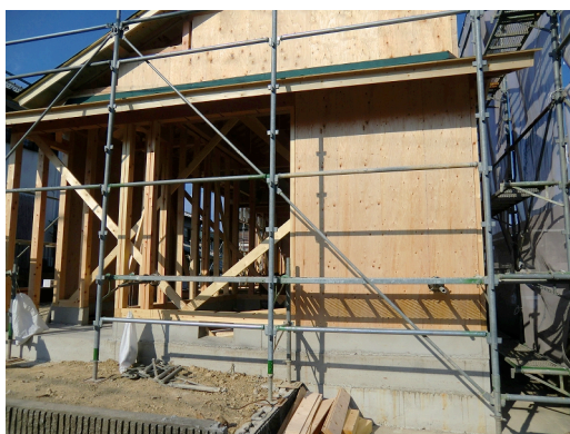
Fig. 2. Structural materials of a building: pillars and walls on the groundwork.
